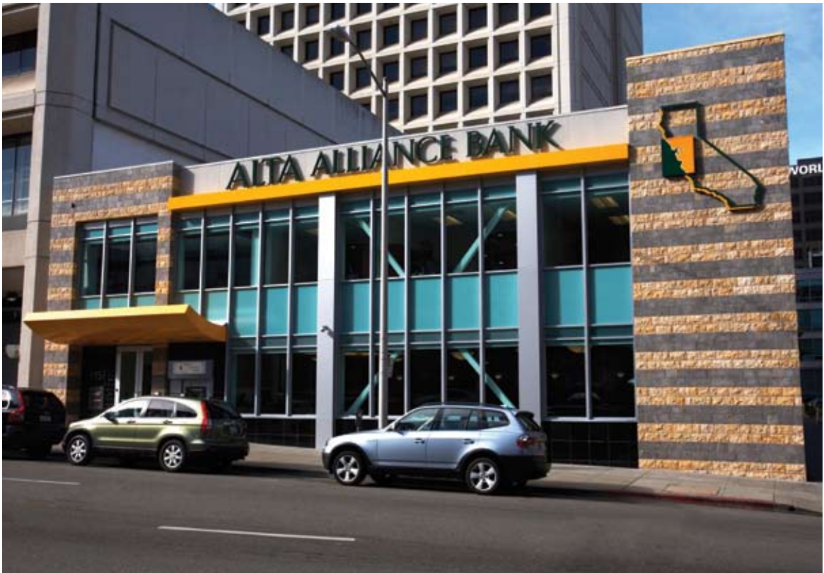
The facade of the 13,000-square-foot Alta Alliance Bank headquarters building, located in Downtown Oakland, CA, features alternating stripes of black and Sand Beige dolomitic limestone in an ashlar pattern, which was added to update the look of the exterior facade.
