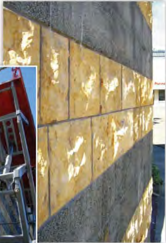
The exterior limestone features a combination of bushhammered and split-faced finishes.
