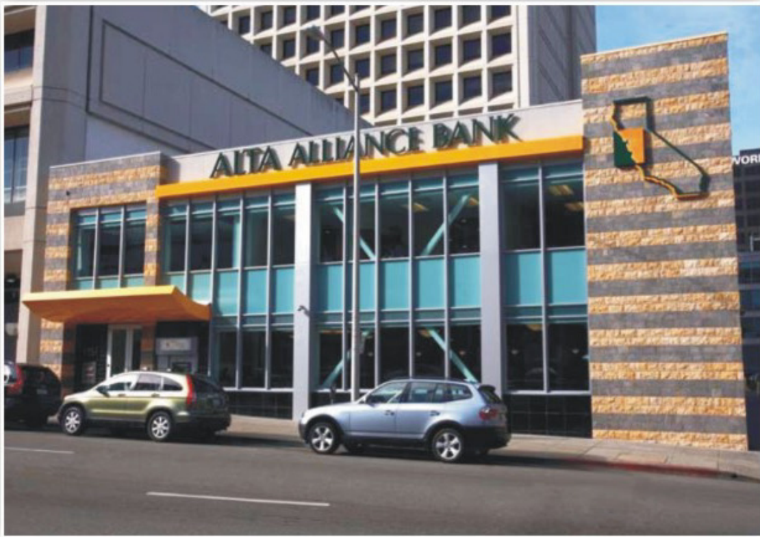
The facade of the 13,000-square-foot Alta Alliance Bank headquarters building, located in Downtown Oakland, CA, features alternating stripes of black and Sand Beige dolomitic limestone in an ashlar pattern, which was added to update the look of the exterior facade.
